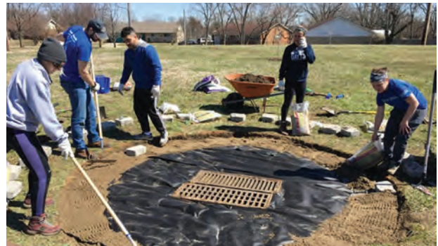
University of Dayton Fitz Center Students Building a Rain Garden at the Madden Hills Community Project. Photo Credit: Fitz Center for Leadership in Community.
