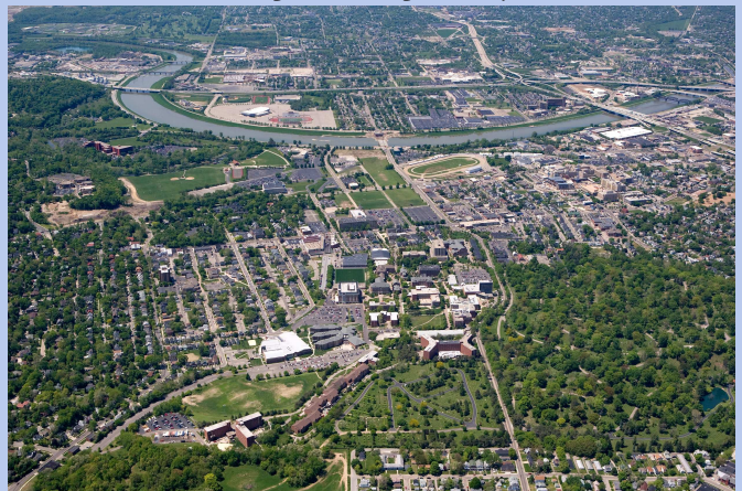
Aerial view of the campus and its proximity to the river.
