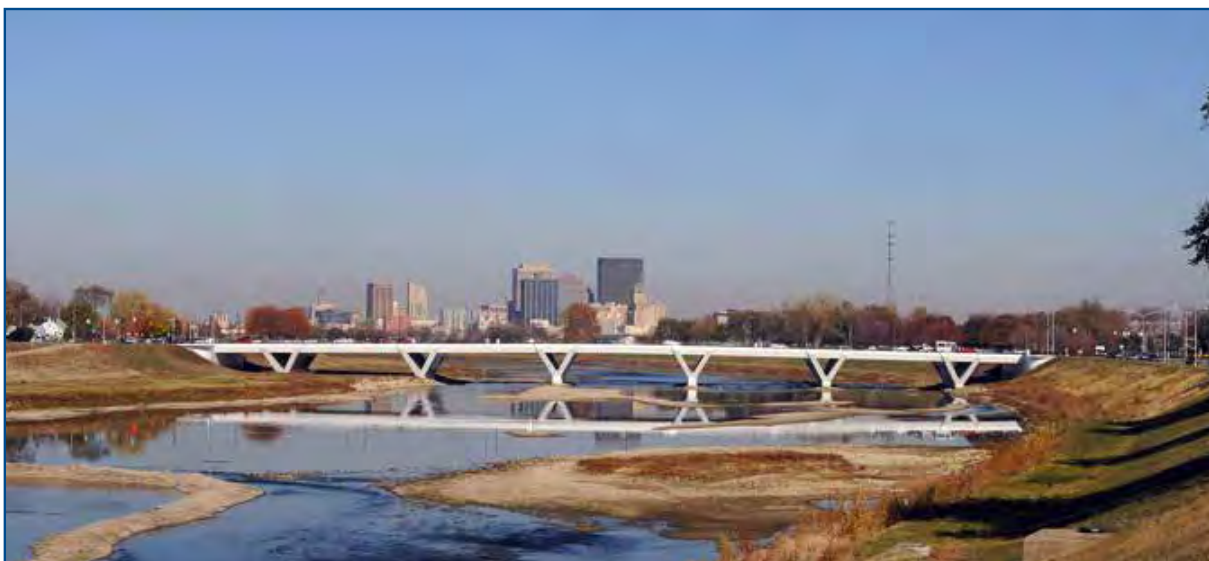
City of Dayton, Ohio, Stewart Street Bridge
