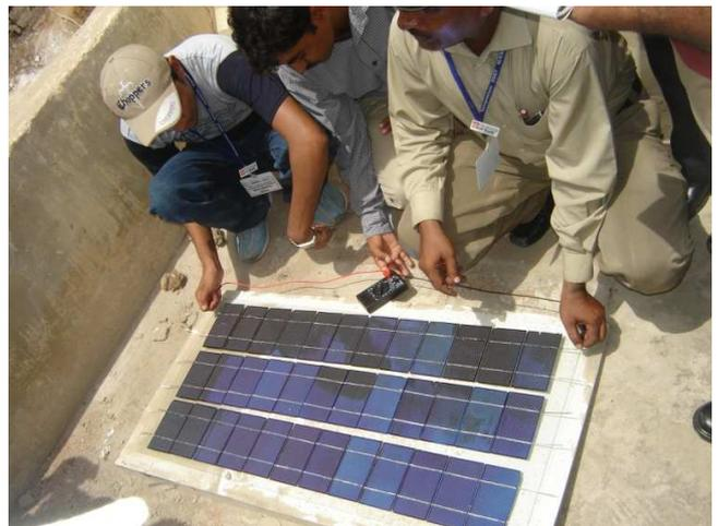
**Figure 2. Testing the voltage and current output of the cell-strings in sunlight**
