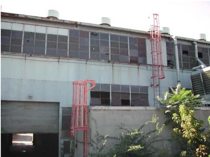
Figure 3. Modern factory with missing, broken and opaque window panes.
