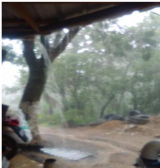
Figure 1: Rainwater spilling over roof without gutters
