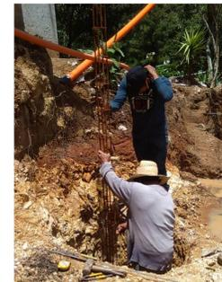
Figure 5: Workers constructing a column to support the kitchen floor
