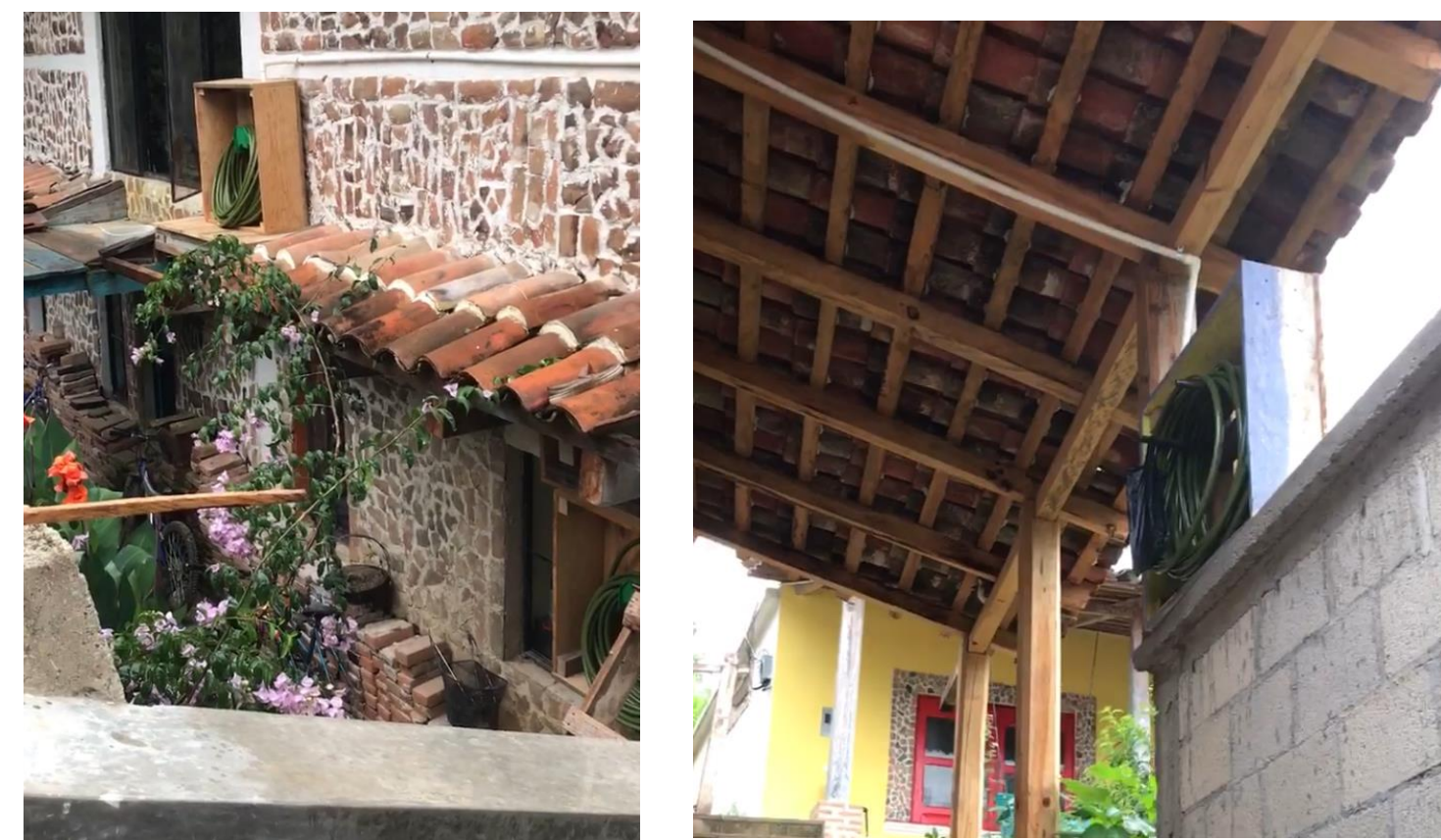
Figures 2 & 3: Three completed hose stations
