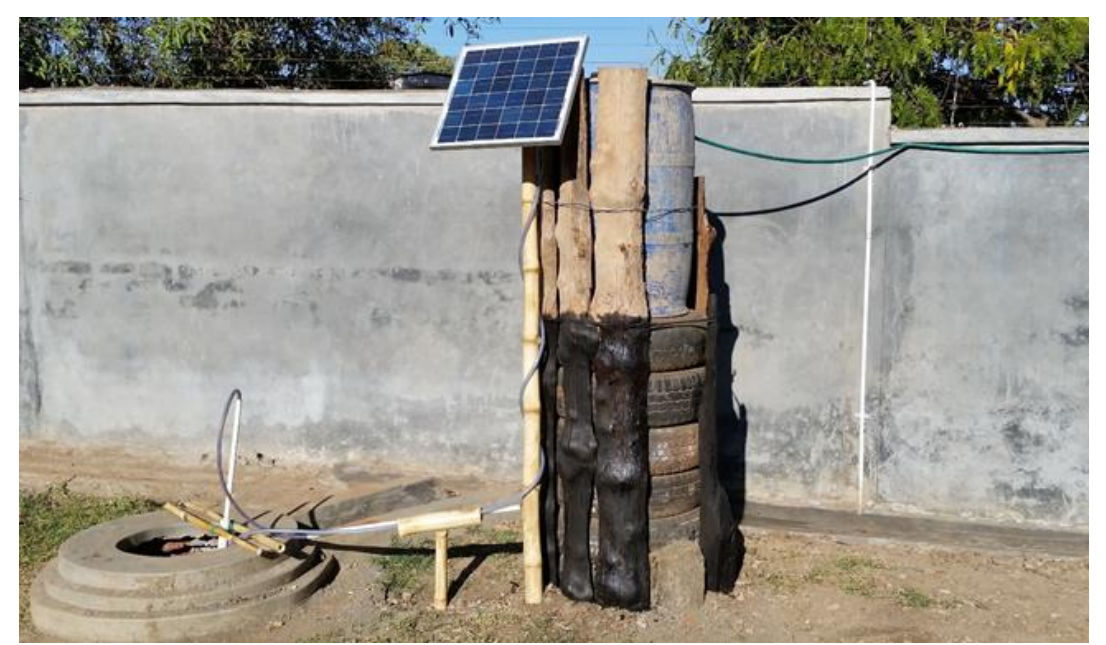
Figure 6: Solar Pump System Assembly
